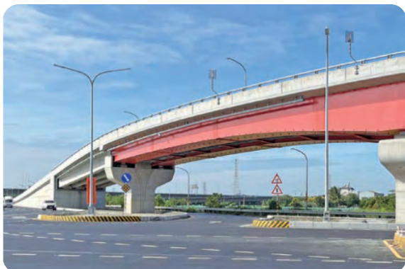
▲ Turn Improvement Project at the Intersection of Xingangshe Boulevard and Nanke Connecting Road
