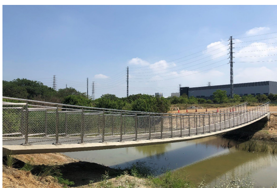
Straight pre-stressed hammock bridge structure
