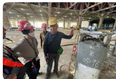
Manufacturing Industry/ TSMC Fab 18 P9 Demolition Project (Counseling of manufacturing industry)
