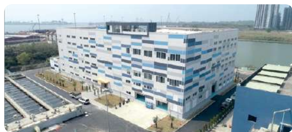
Anping reclaimed water plant
