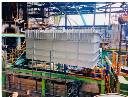
Upgraded Dust Bag Collector for Air Pollution Control and Prevention (2022/09/26)
