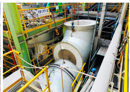
Upgraded Flue Steel Plate and Refractory Materials (2022/10/12)
