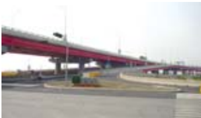
Figure 5-4-6 Southern Access Road
