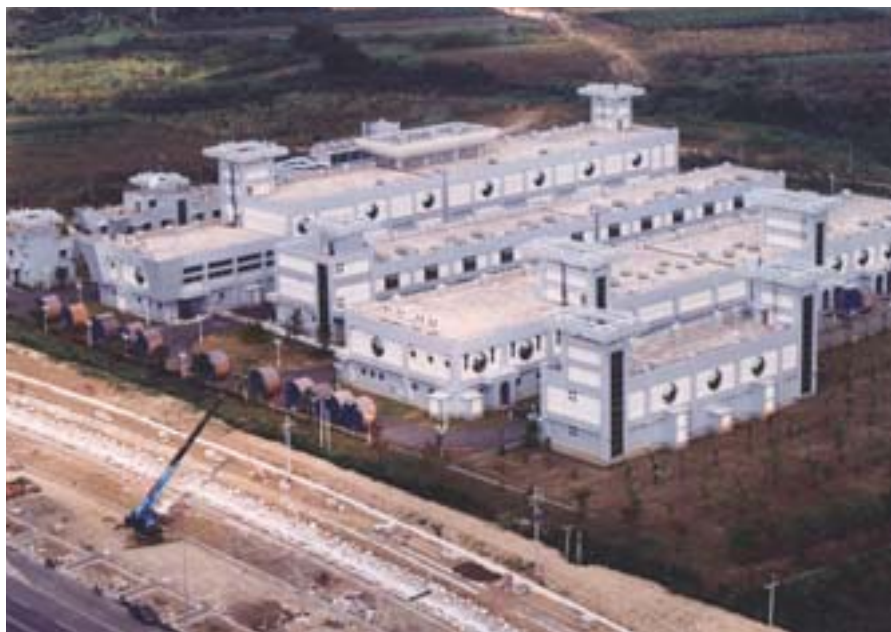
Figure 5-4-3 Extra High Voltage Substation in Tainan Science Park
