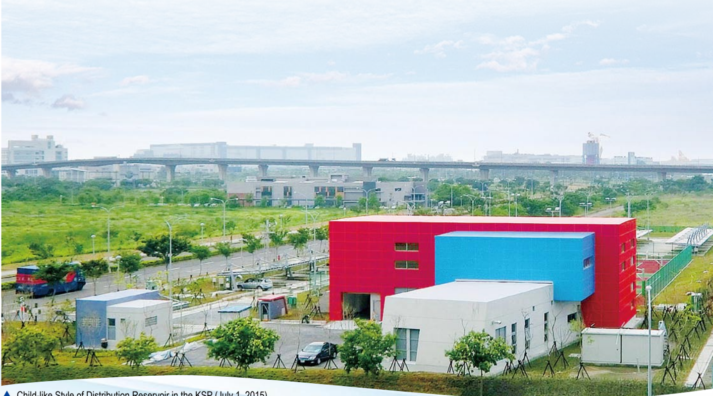
▲ Child-like Style of Distribution Reservoir in the KSP (July 1, 2015)
