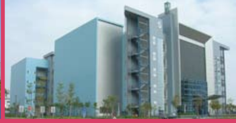
Phase II Standard Factory at the Kaohsiung Science Park
